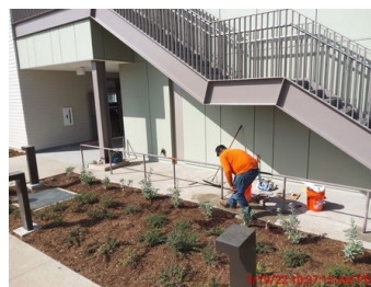
Left to right: Roof finish work, Roof ductwork, 2nd floor landing from staircase # 1 to landscape area, under grand staircase # 2 handrails being installed, under staircase # 1 safety handrail being installed.
