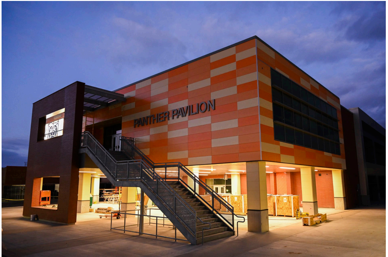
Orange HS – Science Center STEM Building (Dusk with lights)
