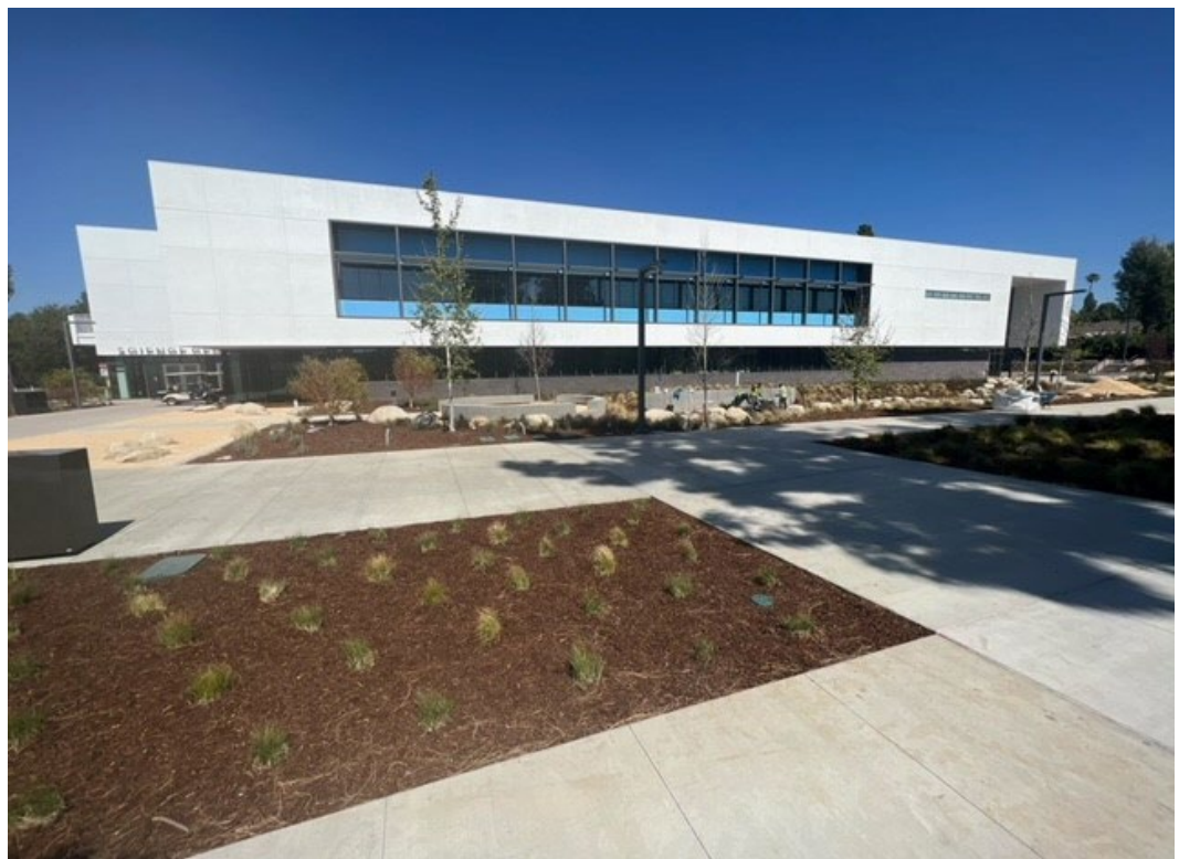
Villa Park HS – Science Center STEM Building (The new Biofiltration area in the foreground next to building)
