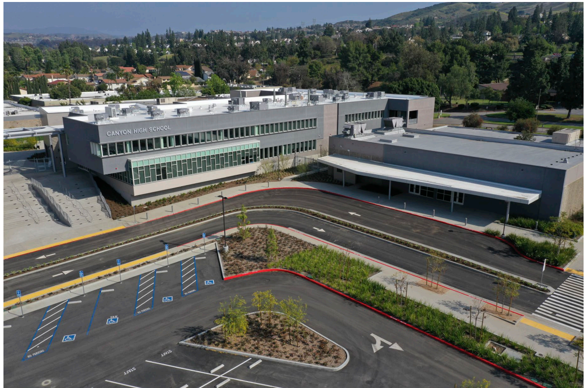
Left to right: Aerial shot of the completed Canyon HS STEM Center (Front of campus, Imperial Hwy view).
