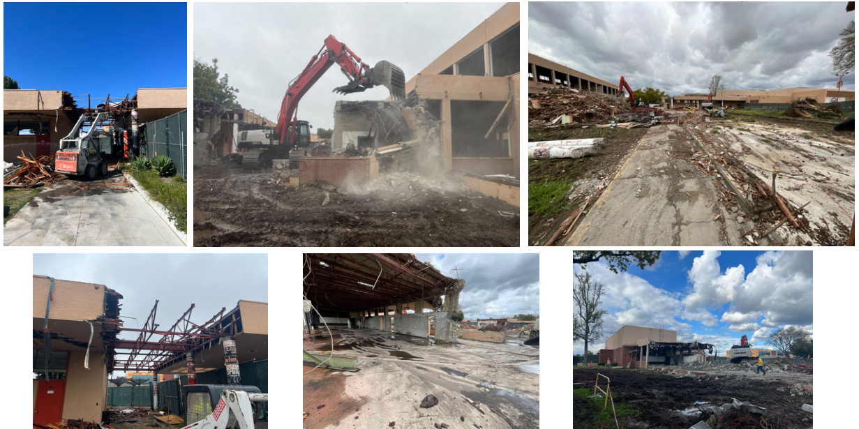
From Top left to bottom right: Construction various demo photos of the building 100/200 interior and exterior.
