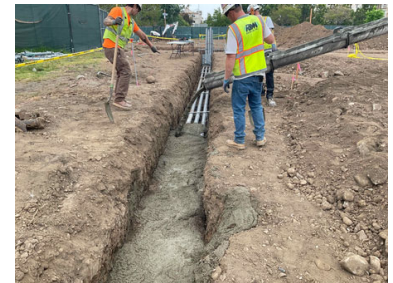
From Top left to bottom right: Construction various excavating and trenching photos of the building 100/200, setting underground conduit and slurry and backfill.
