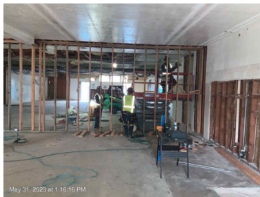
From Top left to bottom right: excavate trenches for the underground plumbing, prepping walls, and floors to run new conduit for electric wiring, exposing ceiling for conduit runs, and interior room demo in Bldg. 800.
