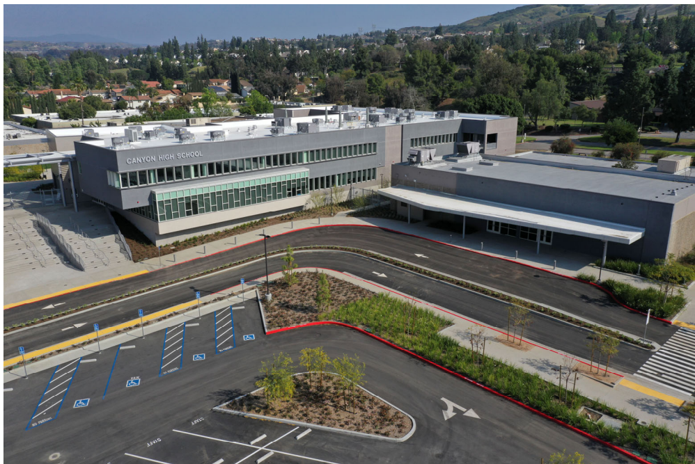
Left to right: Aerial shot of the completed Canyon HS STEM Center (Front of campus, Imperial Hwy view).
