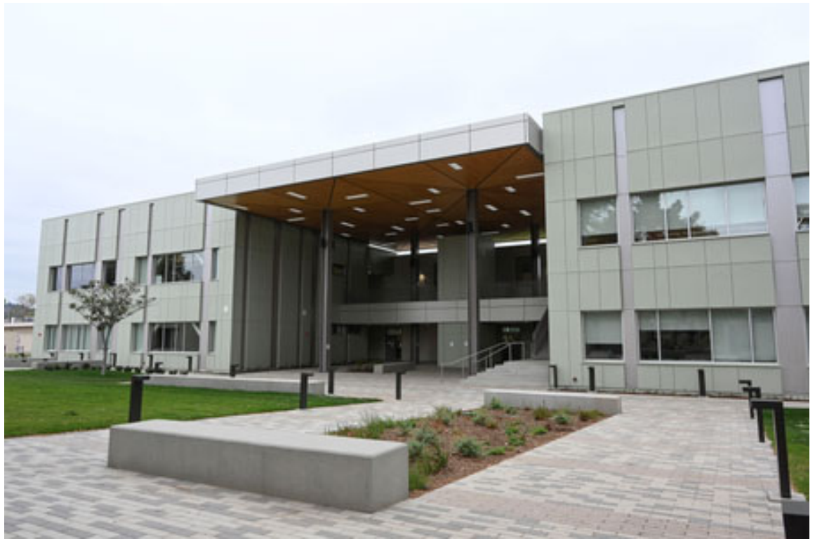
El Modena HS – Science Center STEM Building (Main entrance, facing campus)
