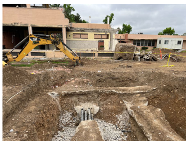
From Top left to bottom right: Construction various excavating and trenching photos of the building 100/200, setting underground conduit and slurry and backfill.
